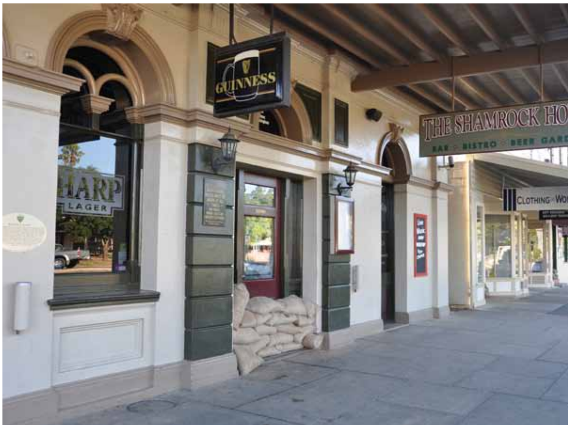
Businesses prepare for floodwaters in Echuca, January 2011. Source: North Central CMA
