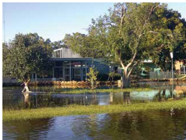
Patients were evacuated as flooding made the Numurkah hospital unusable in March 2012. Source – Moira Shire Council
