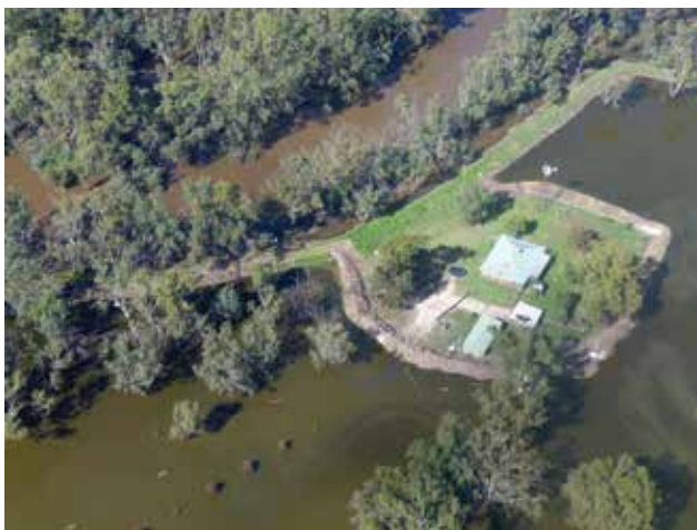
A private levee circling this home kept floodwater out. Source: North Central Catchment Management Authority
