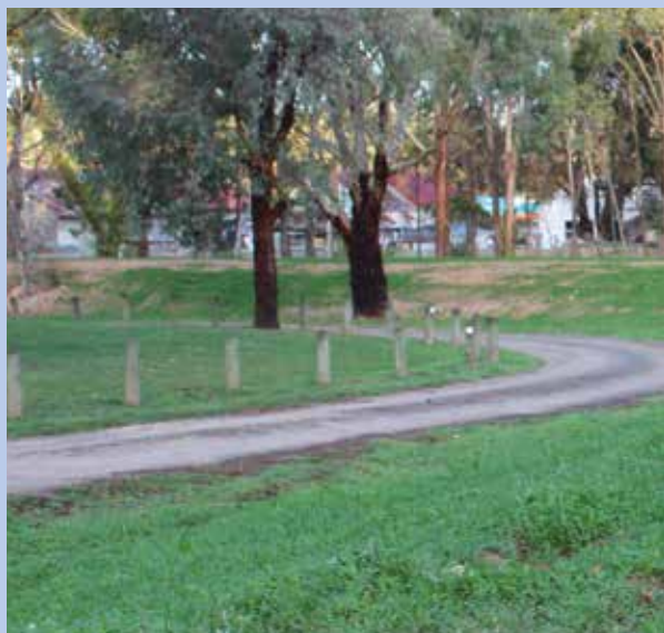
A recently constructed earth levee blends into the landscape of this riverside park in Creswick.
