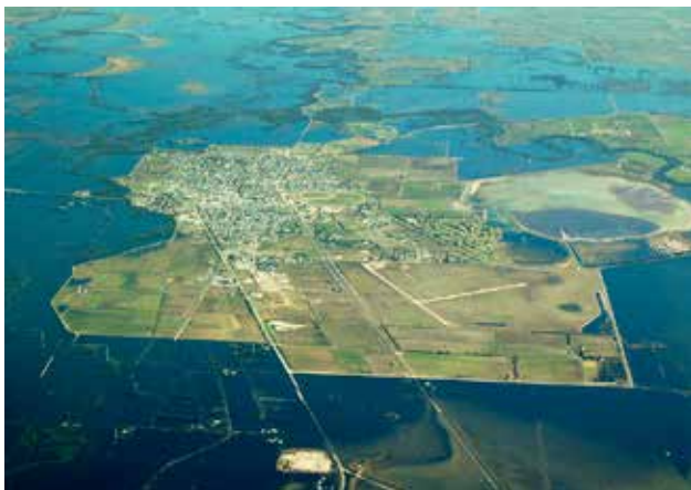
Kerang protected from flood waters by flood mitigation infrastructure. Source: Mallee Catchment Management Authority
